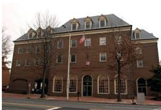
MOAA Headquarters Building Alexandria, now under renovation
